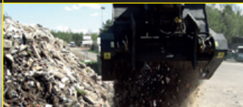
REMUS WL 160HD Mixcross grävmaskin, schakt porslin tegel, sten, betong
